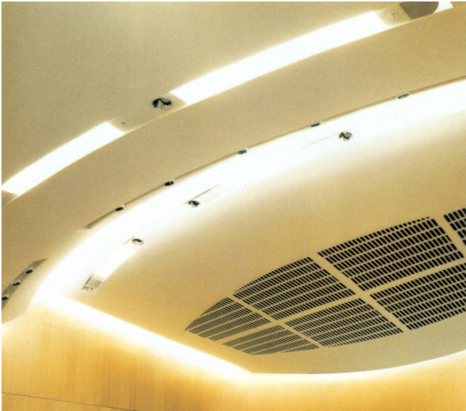
GENERAL VIEW OF CEILING
