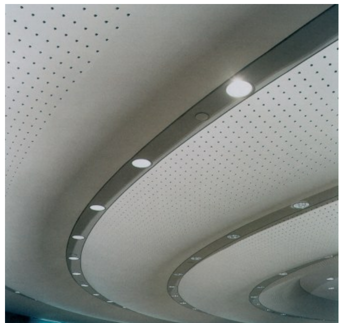
DETAIL OF CURVED CEILING
