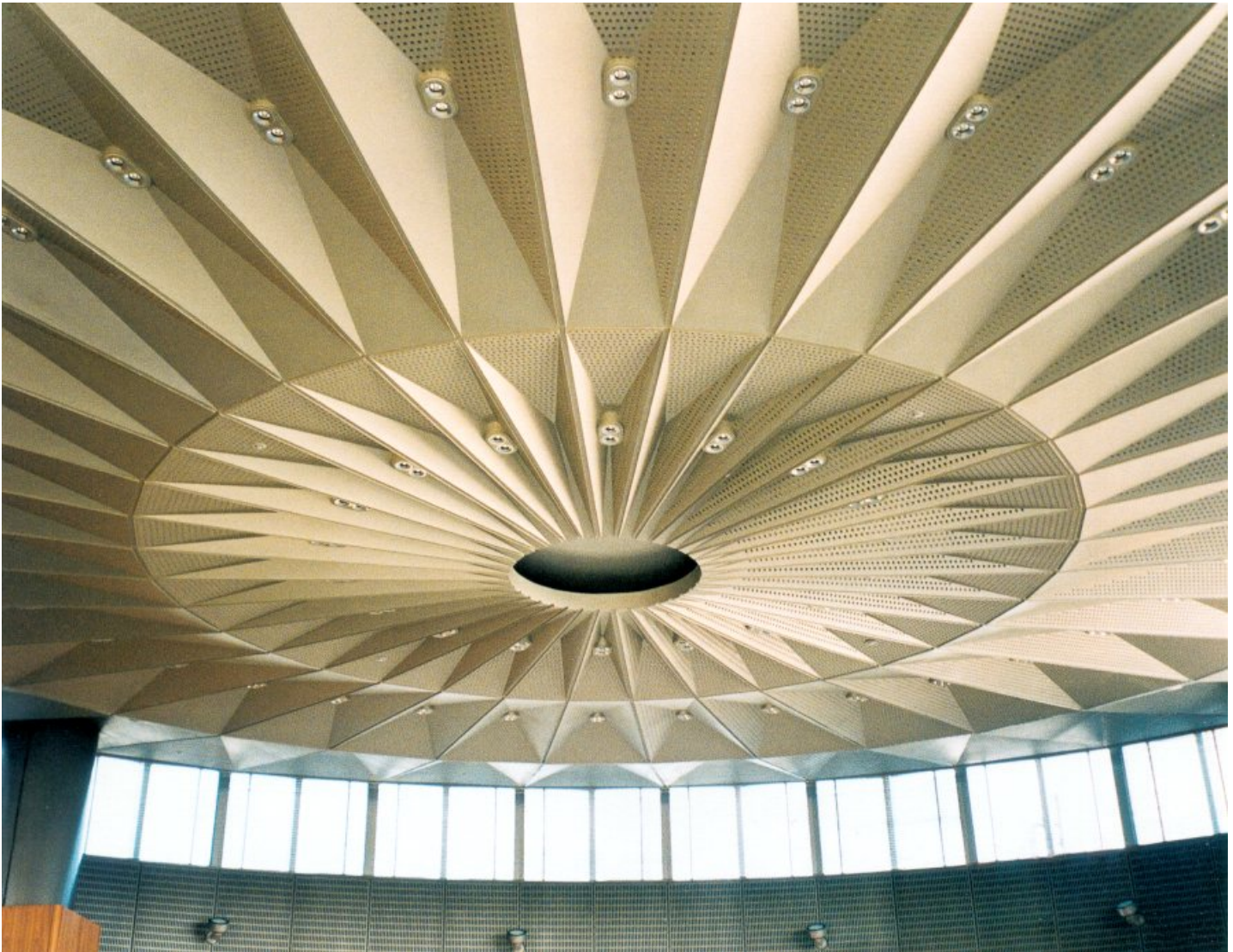
LECTURE HALL CEILING
